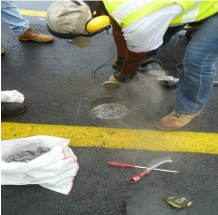
Angle grinder is used to mark out area
