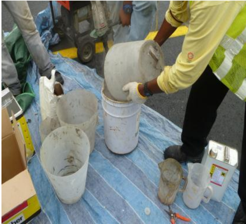
Filler component is then added to the mixed Resin and Activator
