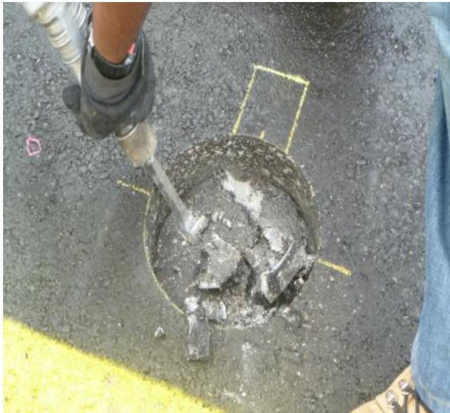
A jack hammer is used to break out the concrete and expose the cables
