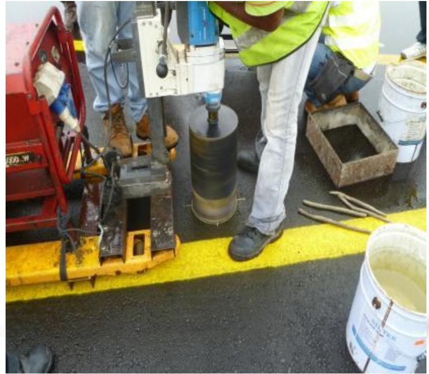
A metal case is placed in position and sealed to allow wet coring
