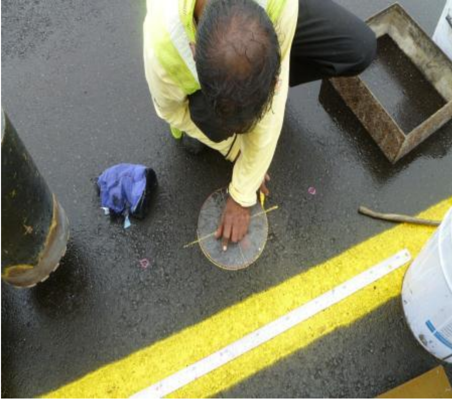
The diameter of the core hole is clearly set out
