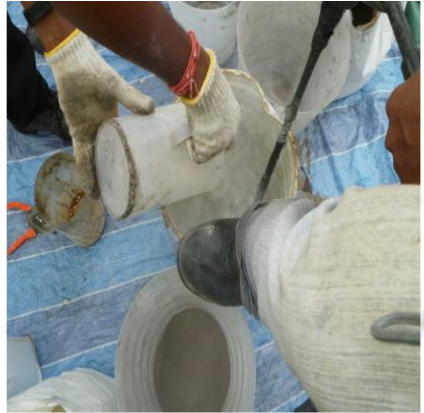
Activator is then added to the Resin and mixed with a slow speed drill for approximately 1 minute
