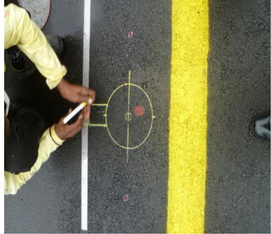
The lug is set out and adjacent core marking
