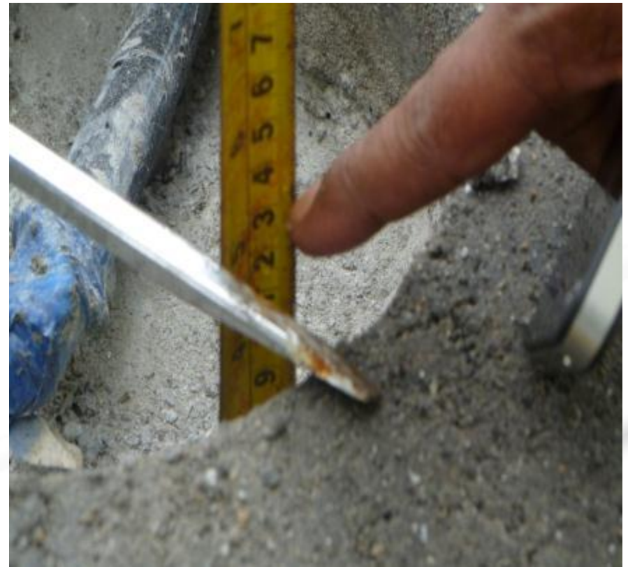
Cable is exposed and depth measurement is taken
