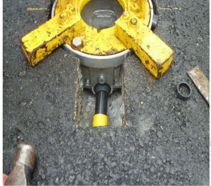
The cable is then connected to the base and placed in position with the jacks note the gap under the base
