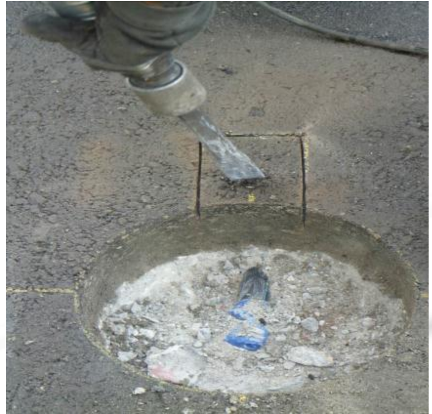
A jack hammer is used to break out the asphalt
