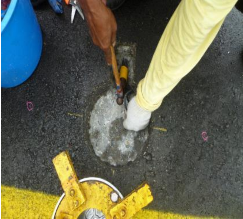
A ridged connector is fitted to cable
