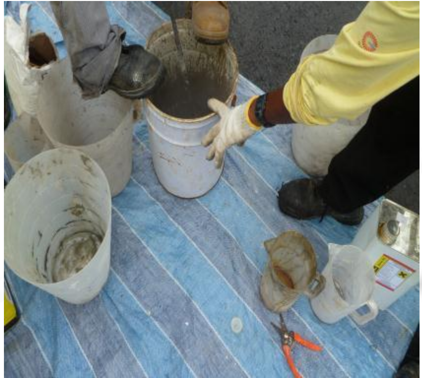
Filler component is then mixed to the Resin and Activator
