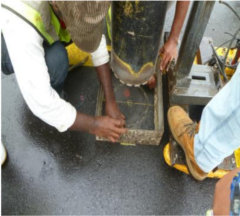
Initial coring to mark out the core diameter
