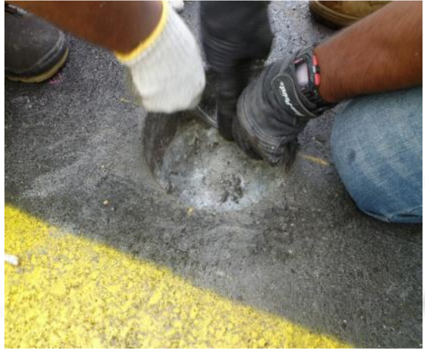
The cable rope is then pulled through
