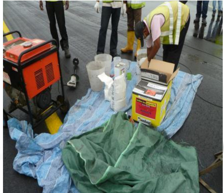
Components are placed on a ground sheets during mixing to protect the asphalt surface from spillage
