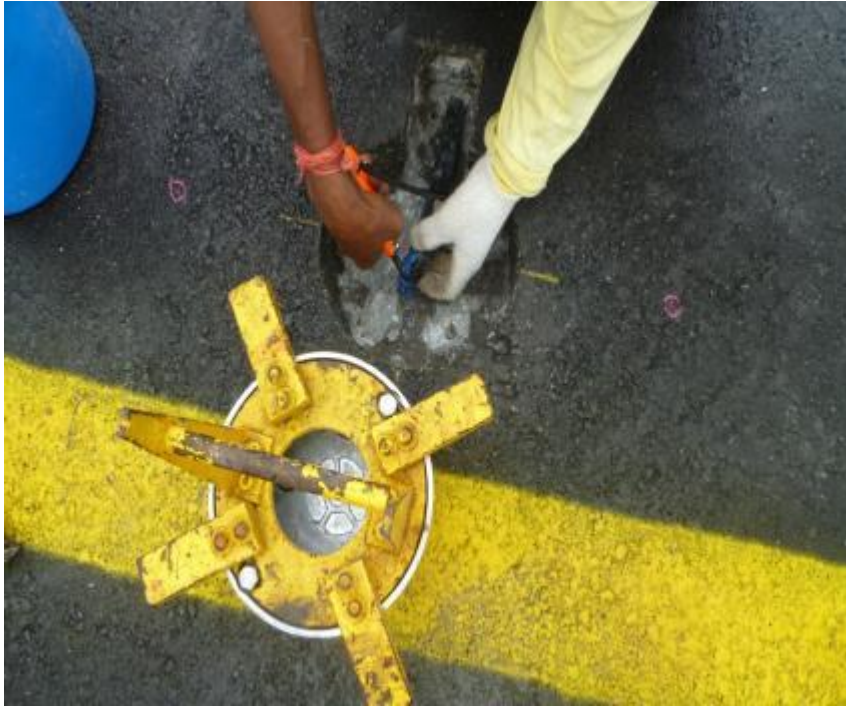
The tape protecting the cable end is cut
